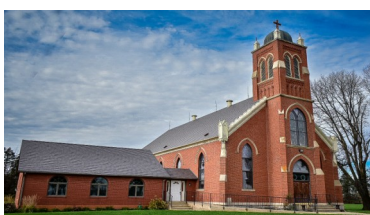
St. Columbkil Church (SC) 36483 County 47 Boulevard Goodhue, MN 55027
